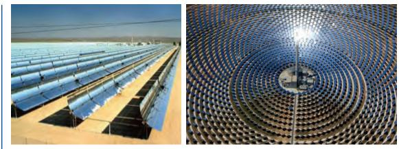
Parabolic Trough Concentrating Solar Collector at Kramer Junction, California Source: NREL 2012a
